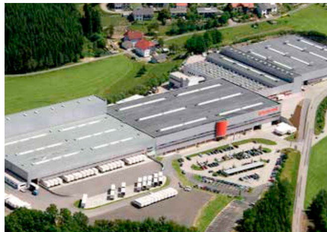
SARLEINSBACH/UPPER AUSTRIA UPVC window and insulating glass production, extrusion
