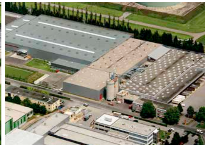
LANNACH/STYRIA Timber/aluminium production
