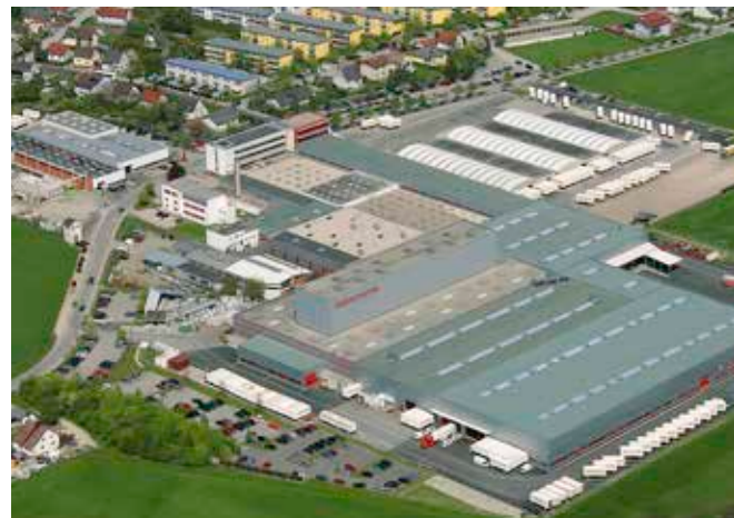
TRAUN/UPPER AUSTRIA UPVC window, insulating glass and aluminium production
