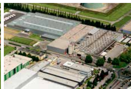
Lannach/Styria Timber/aluminium production
