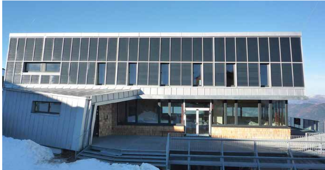
Ludwig Walter House/Carinthia: Dobratsch Summit House at 2143 m altitude. Architect DI Weratschnig, Transform Architekten ZT-GmbH
