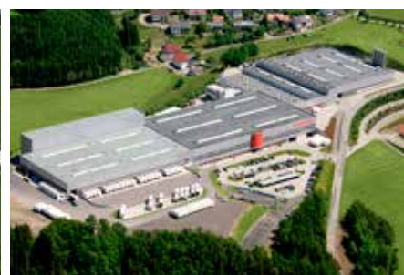
Sarleinsbach/Upper Austria UPVC window and insulating glass production, extrusion
