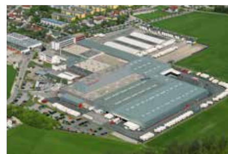
Traun/Upper Austria UPVC window, insulating glass and aluminium production
